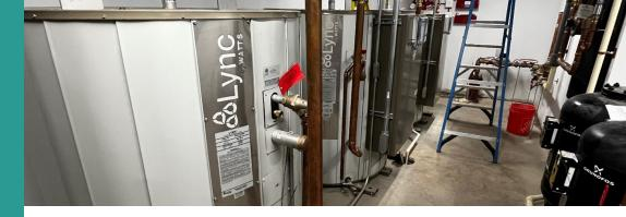
backup heating. Not only does Aegis operate at lower ambient temperatures than many alternative solutions, but it also maintains the ability to deliver hot water well above 140°F when the weather turns colder. CO<sub>2</sub> refrigerant also exceeds expectations when compared to other common refrigerants used in heat pump water heaters with a Global Warming Potential (GWP) of 1.
